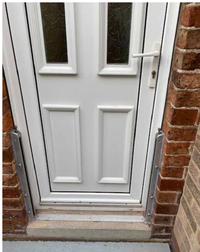
Above: Support brackets for flood barrier installed
